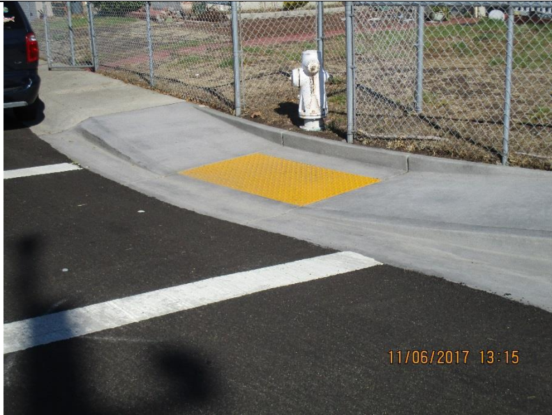
UPGRADED CURB RAMP AT PURDUE-ESSER
