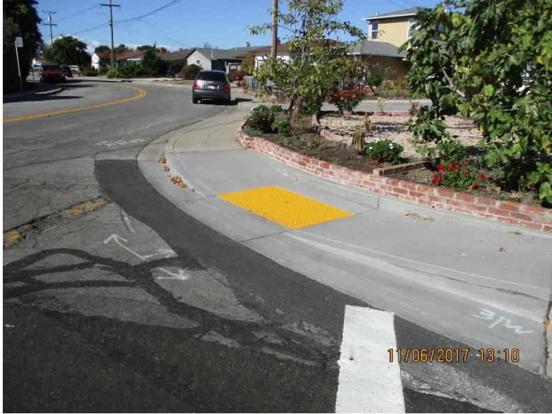
UPGRADED CURB RAMP AT BURKHART-LAVERNA
